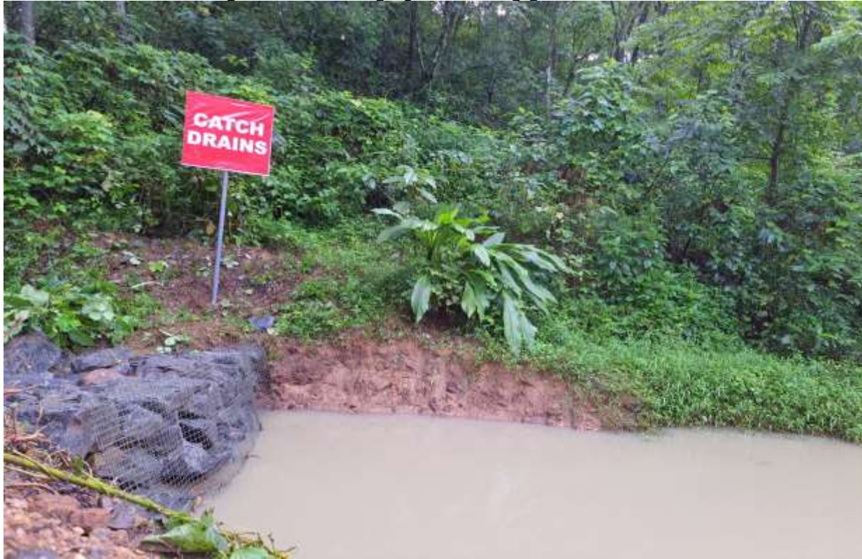
Figure I0 : Photographs showing garland drains
