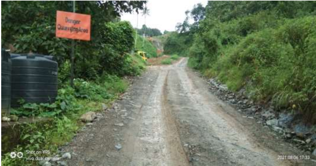
Figure 7: Photograph showing access road to the project area
