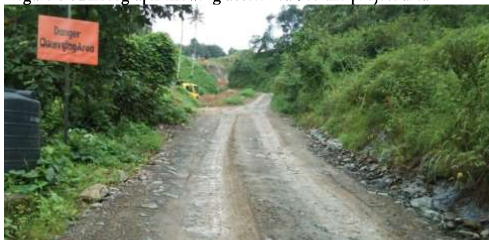
Figure 3 : Photograph showing access road to the project area
