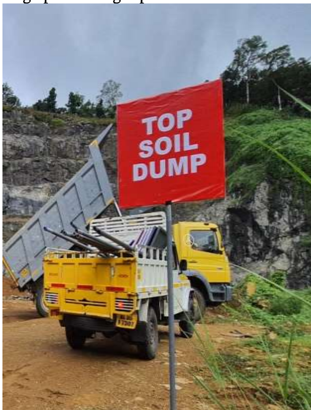
Figure I : Photograph showing top soil and overburden in the project site
