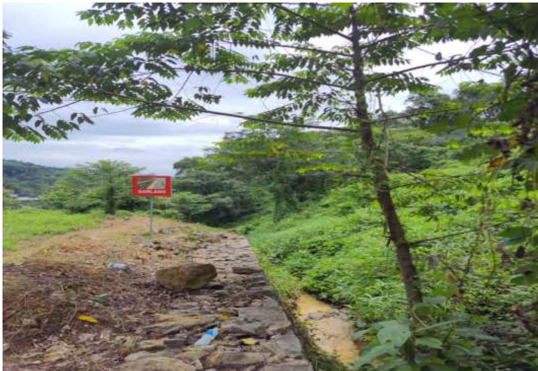
Figure 2 : Photographs showing garland drains
